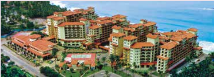
Marbella Hotel, Condominium
